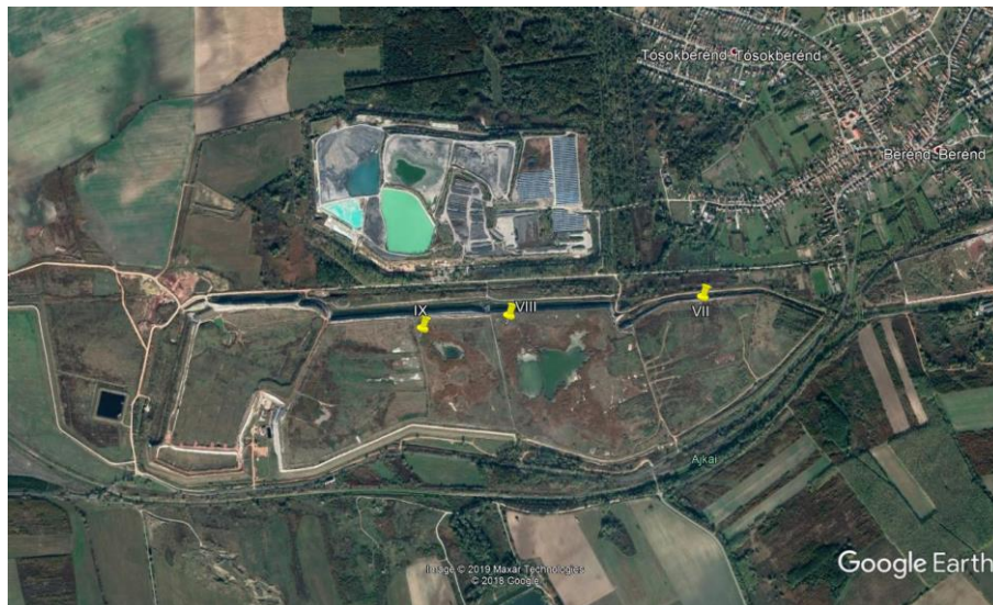
Figure 10C. Aerial view of Ajka red mud landfill with indication of drilling positions along red mud accumulation cells No. VII., VIII. and IX.
