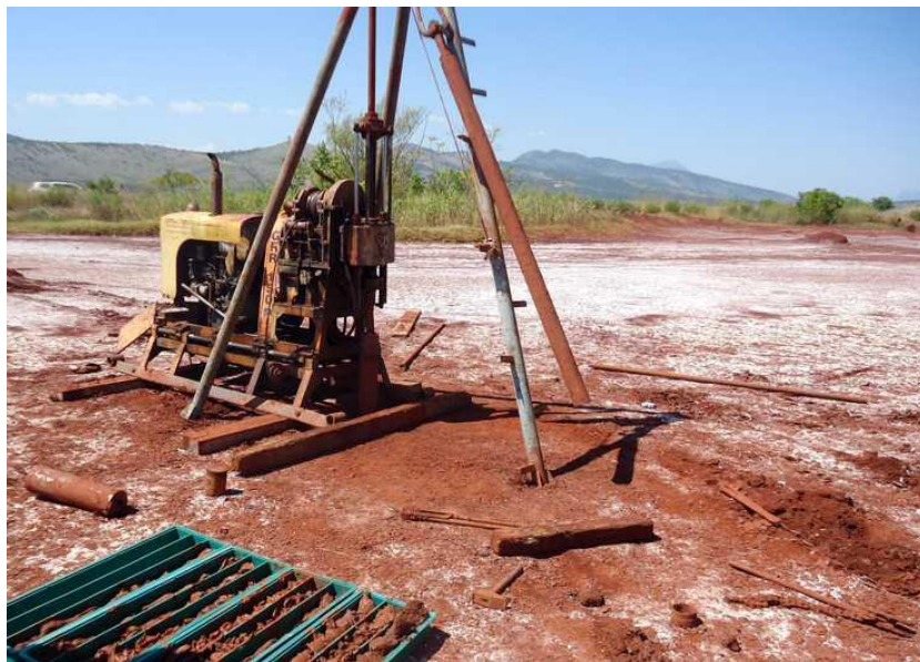
Figure 10B. Drilling activities in the red mud landfill near Podgorica within WP3 tasks
